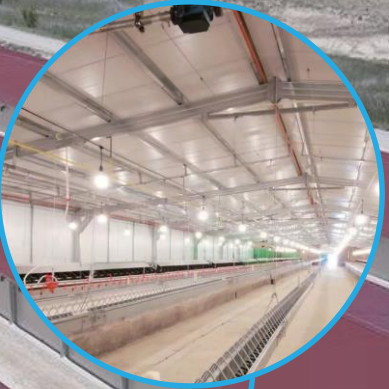
Feeding line hoisting
